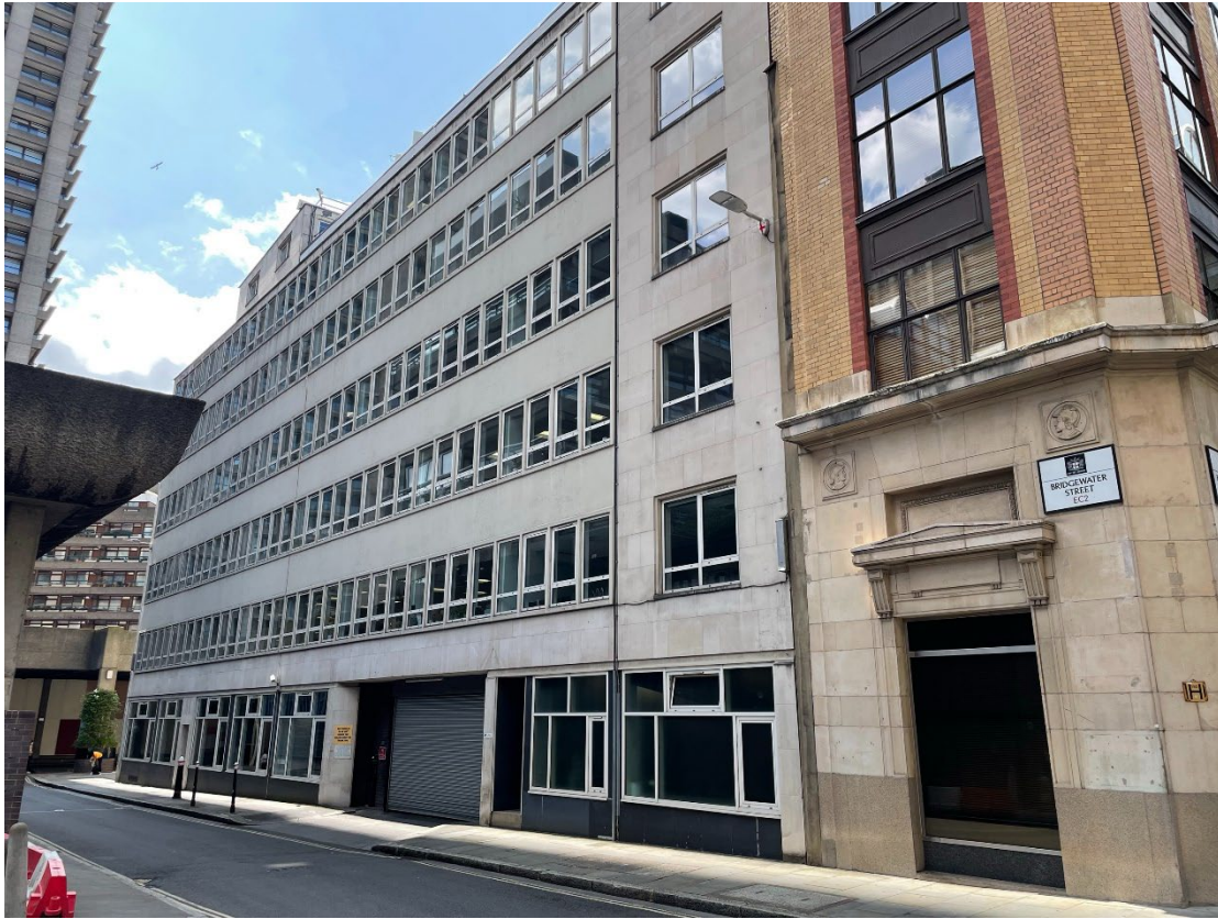
Image 3: View of Bridgewater Street elevation
