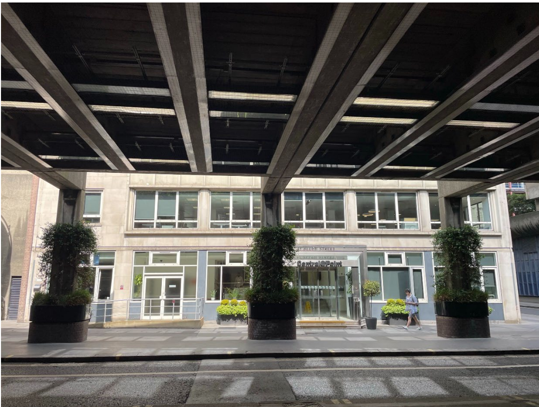
Image 2: View of front elevation taken from Beech Street tunnel.
